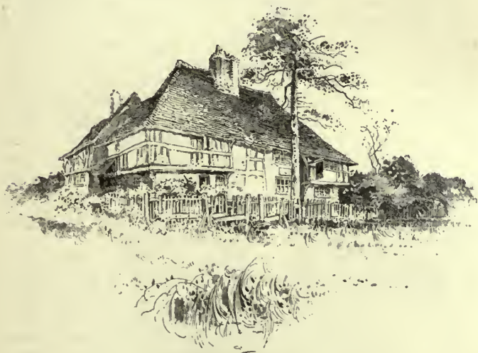
A Roadside Inn, Hollingbourne.
